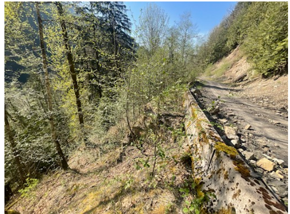
Grs wall on mse stacked rocks.
